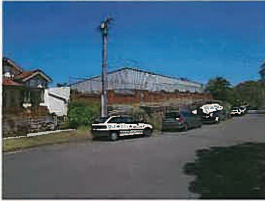
Figure 3: Existing reservoir structure, looking southwest from Fairlight Street (Photograph dated 23 rd October 2013)
