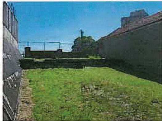
Figure 6: Eastern side of existing reservoir structure, looking north (Photograph dated 23 rd October 2013)
