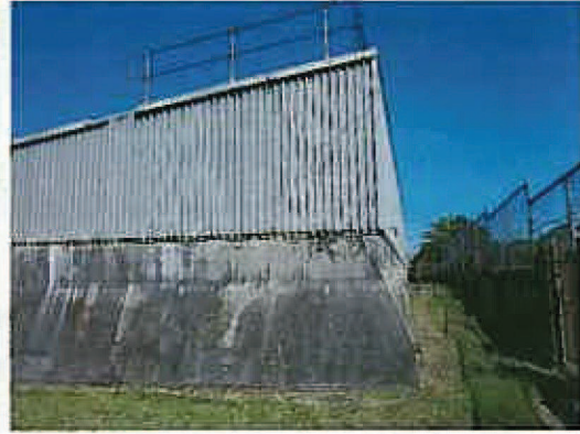
Figure 4: Existing reservoir structure, looking west from northeast corner of structure (Photograph dated 23 rd October 2013)
